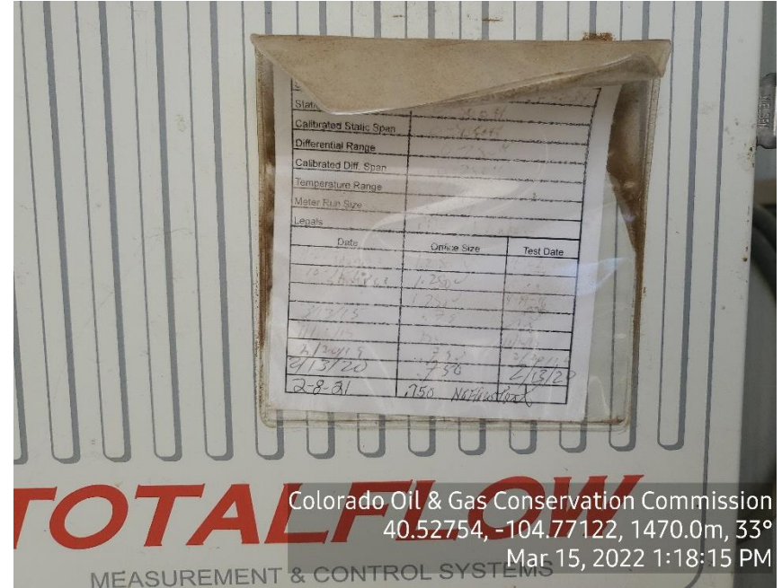
Photo 6: Gas meter not calibrated annually
