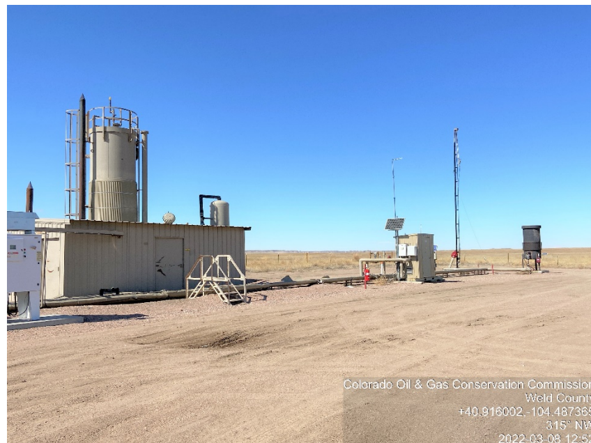
Photo #4 Lion Creek 02-13 Battery site Inactive / Shut-down Treater, Separator, ECD
