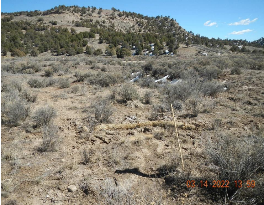
Wattle along flow path of Spill/Release Point ID #481666.
