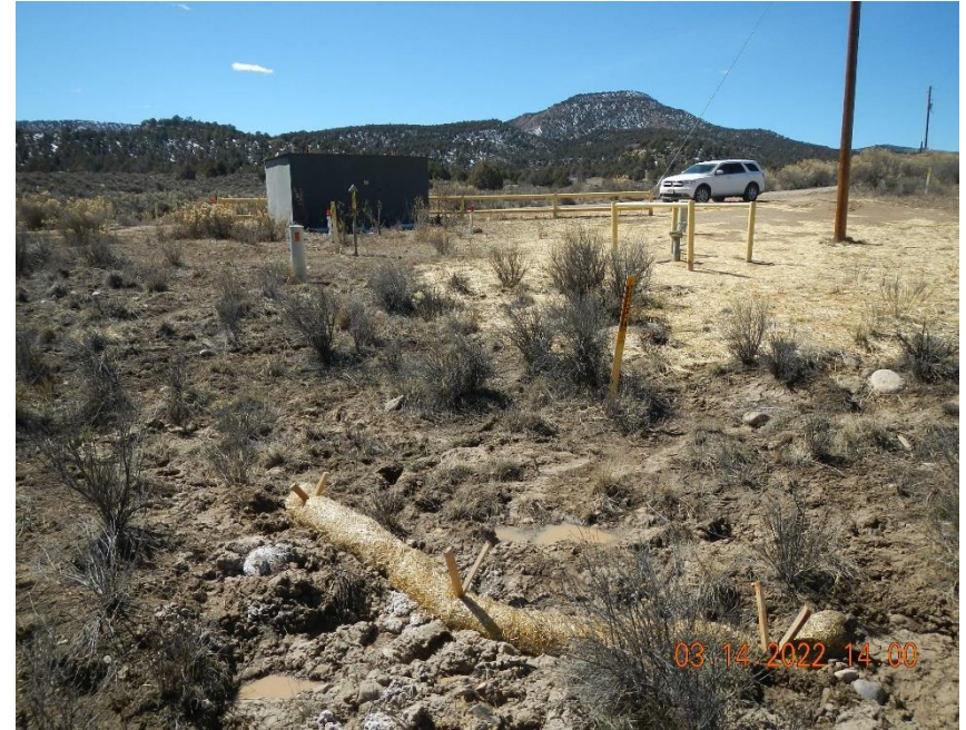
Wattle downstream of release point.
