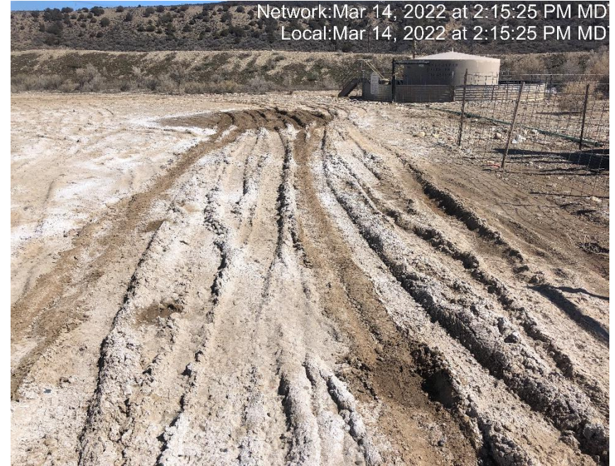
Photo #6167 Location lacks stabilization.
