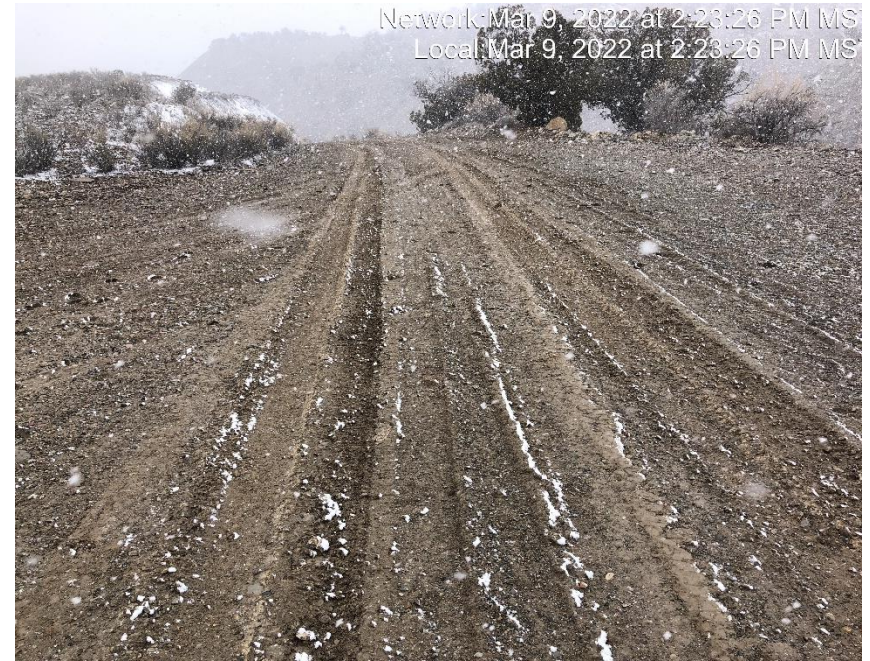
Photo #6129 Insufficient tracking control located at the entrance to location.
