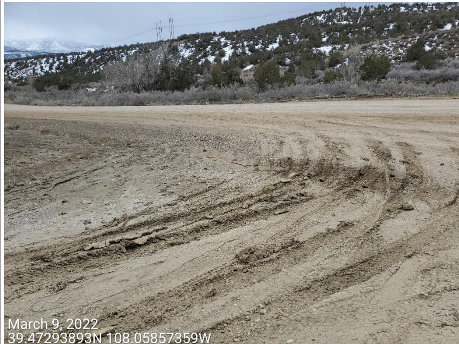
Photo 1: Photos taken from the access road (photo left access road turn off). Photos examples showing control measures / BMPs to stabilize the access road, minimize tracking and offsite sediment transport are missing or insufficient.
