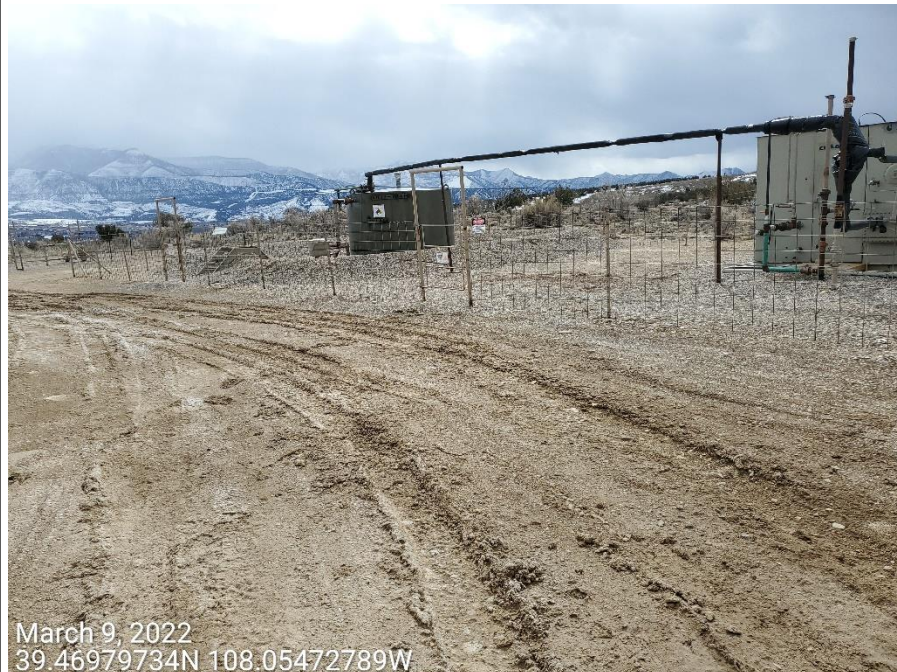
Photo 3: Photos taken from the Location. Photos examples showing control measures / BMPs to stabilize the Location, minimize tracking and offsite sediment transport are missing or insufficient.
