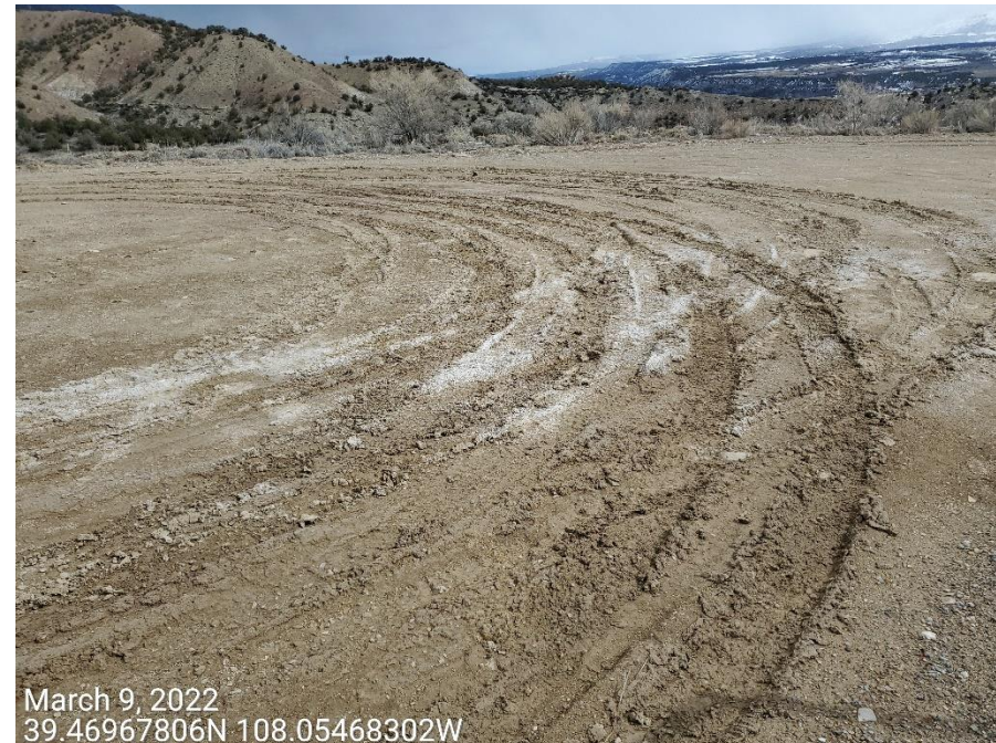
Photo 3: Photos taken from the Location. Photos examples showing control measures / BMPs to stabilize the Location, minimize tracking and offsite sediment transport are missing or insufficient.
