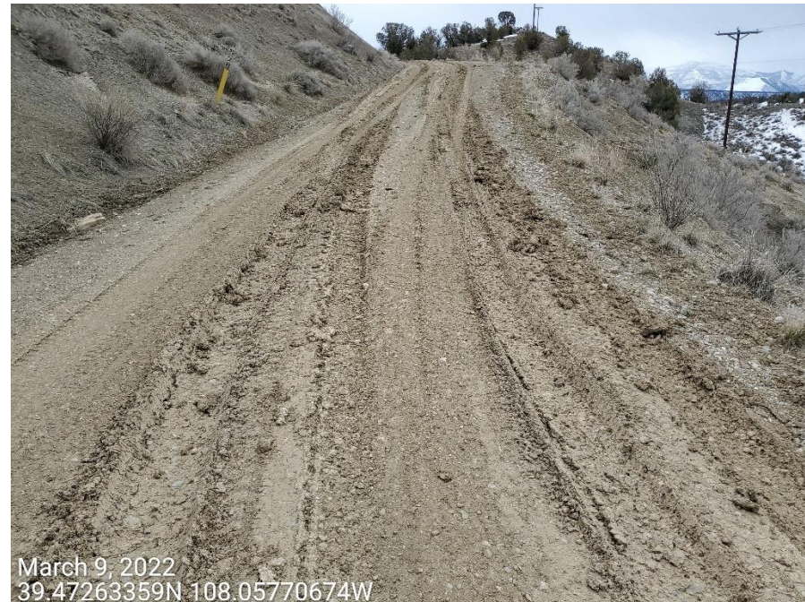
Photo 1: Photos taken from the access road (photo left access road turn off). Photos examples showing control measures / BMPs to stabilize the access road, minimize tracking and offsite sediment transport are missing or insufficient.
