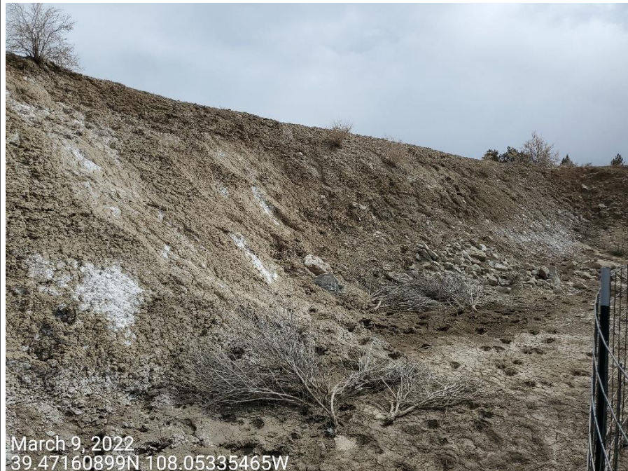
Photo 2: Photos 2-3 taken from the cut slopes on the east and southern ends of the Location. Photos show control measures are missing or insufficient to protect/stabilize the cut slopes.
