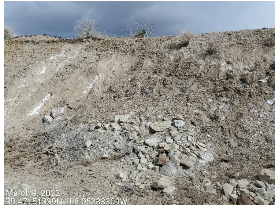
Photo 2: Photos 2-3 taken from the cut slopes on the east and southern ends of the Location. Photos show control measures are missing or insufficient to protect/stabilize the cut slopes.
