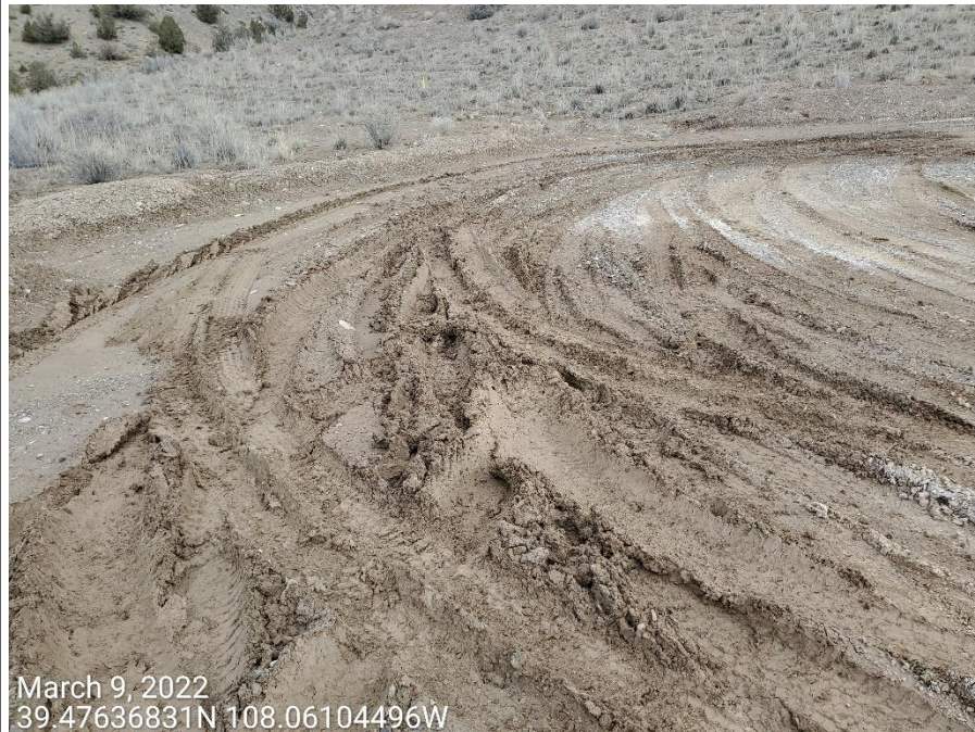
Photo 2: Photos taken from the Location. Photos examples showing control measures / BMPs to stabilize and minimize tracking/sediment transport from the road and Location remains missing or insufficient.
