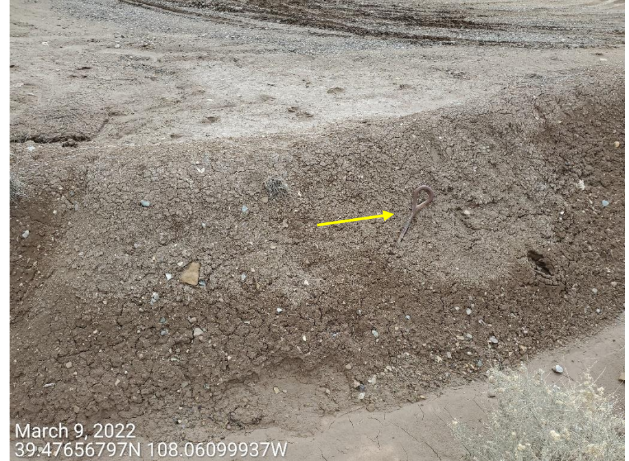
Photo 4: Photos examples showing markers at anchors on Location are missing, or in disrepair.
