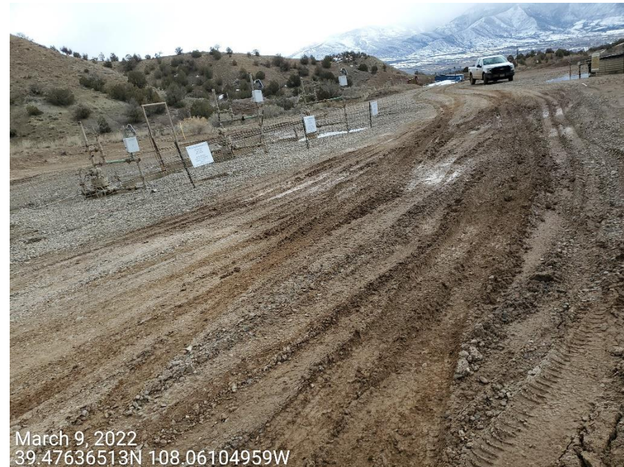
Photo 2: Photos taken from the Location. Photos examples showing control measures / BMPs to stabilize and minimize tracking/sediment transport from the road and Location remains missing or insufficient.
