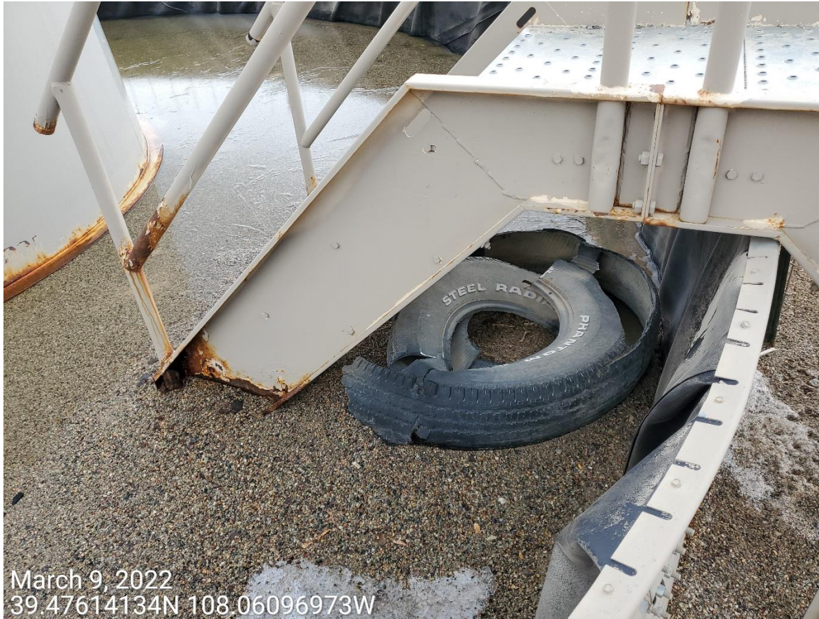
Photo 5: Photo shows trash debris improperly stored within the secondary containment of the tank battery.
