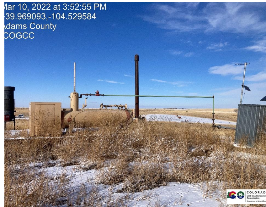
Pic 6 ECD, Separator, Gas meter run, weeds unmanaged on location.
