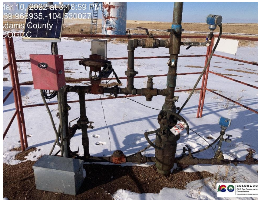
Pic 1 wellhead, All flowline valves, and master valve are in the close position. One flowline off of the top of the lubricator is seized slightly open. Flowlines downstream of valve are in the close position. Stained soil by wellhead.
