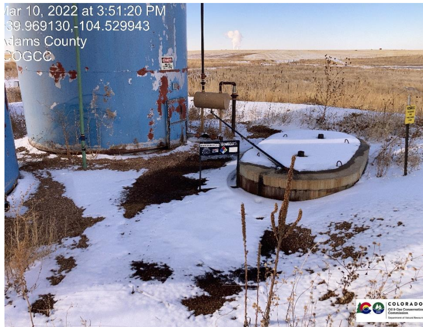
Pic 5 Stained soil around water tank, spill was never cleaned up from previous inspections. Water tank, and 1 oil tank appear to have fluid in them.
