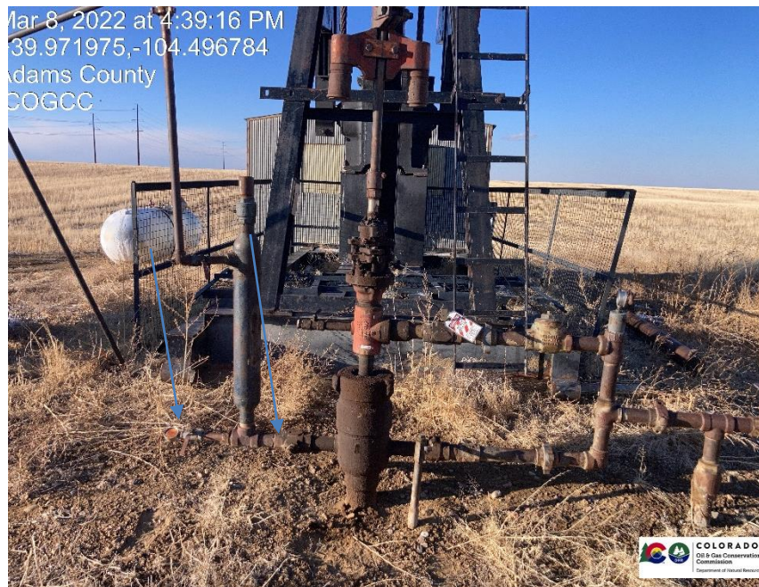
Pic 1 Casing valve is venting gas. 2" ball valve is seized slightly open, and the ½" ball valve has a crack in the back of the valve that is venting gas. All other valves are in the close position.
