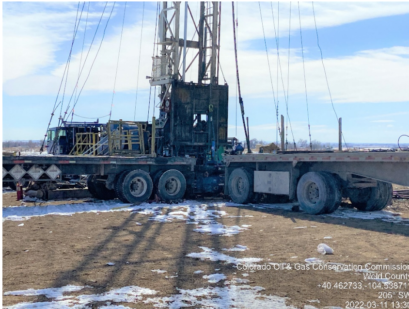
Photo #1 Howard 3-27 (05-123-13811) Wellsite Shut-In | SI Plugging Operations: Bleed down | WK Bleed down well, prep for plugging.
