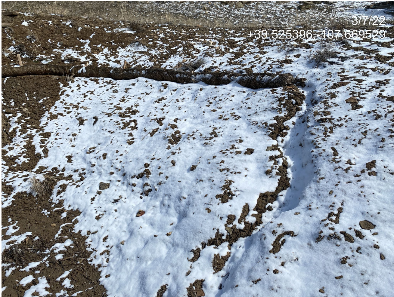
Photo 3. Photo taken from the north of the location shows rill erosion occurring on cut slopes.
