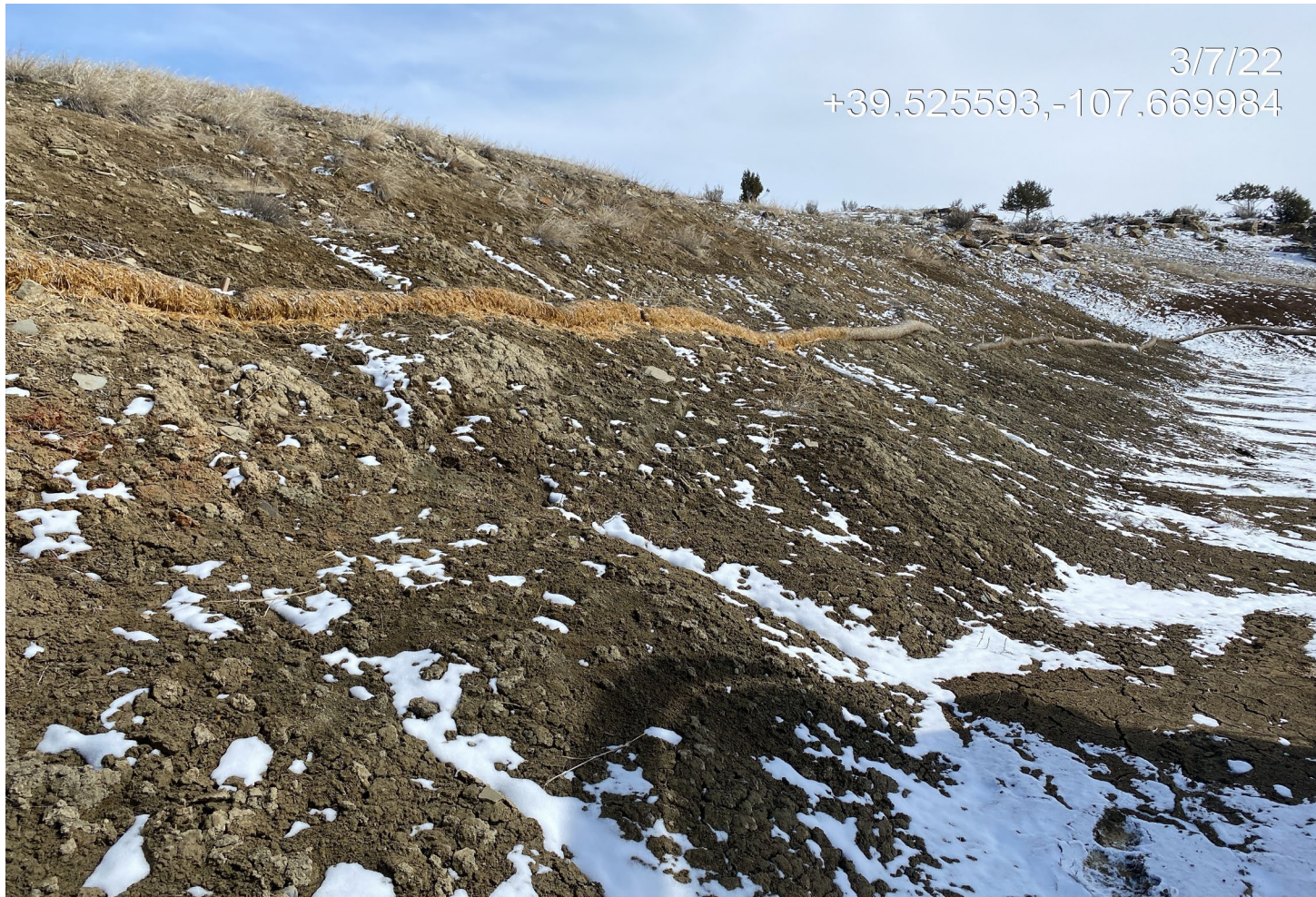
Photo 1. Photo taken from the north of the location facing east shows rill erosion occurring on cut slopes.
