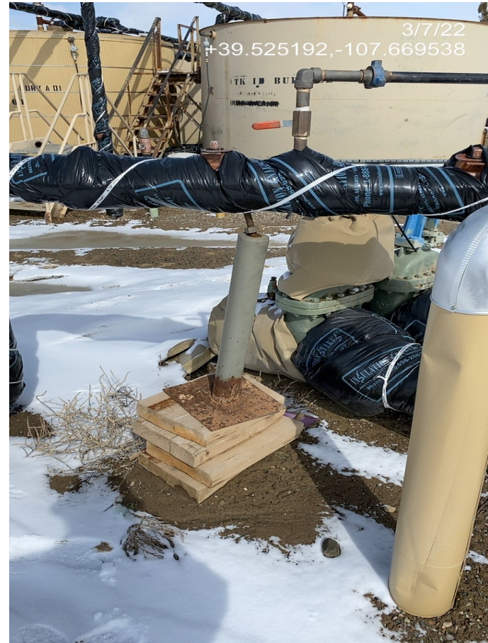
Photo 6. Photo taken from the southeast of the location shows a support beam that is not in proper functioning condition.
