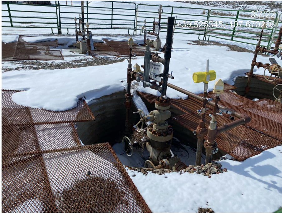
Photo 8. Photo taken at the well location shows wildlife protection control measures on well cellar are not properly installed.
