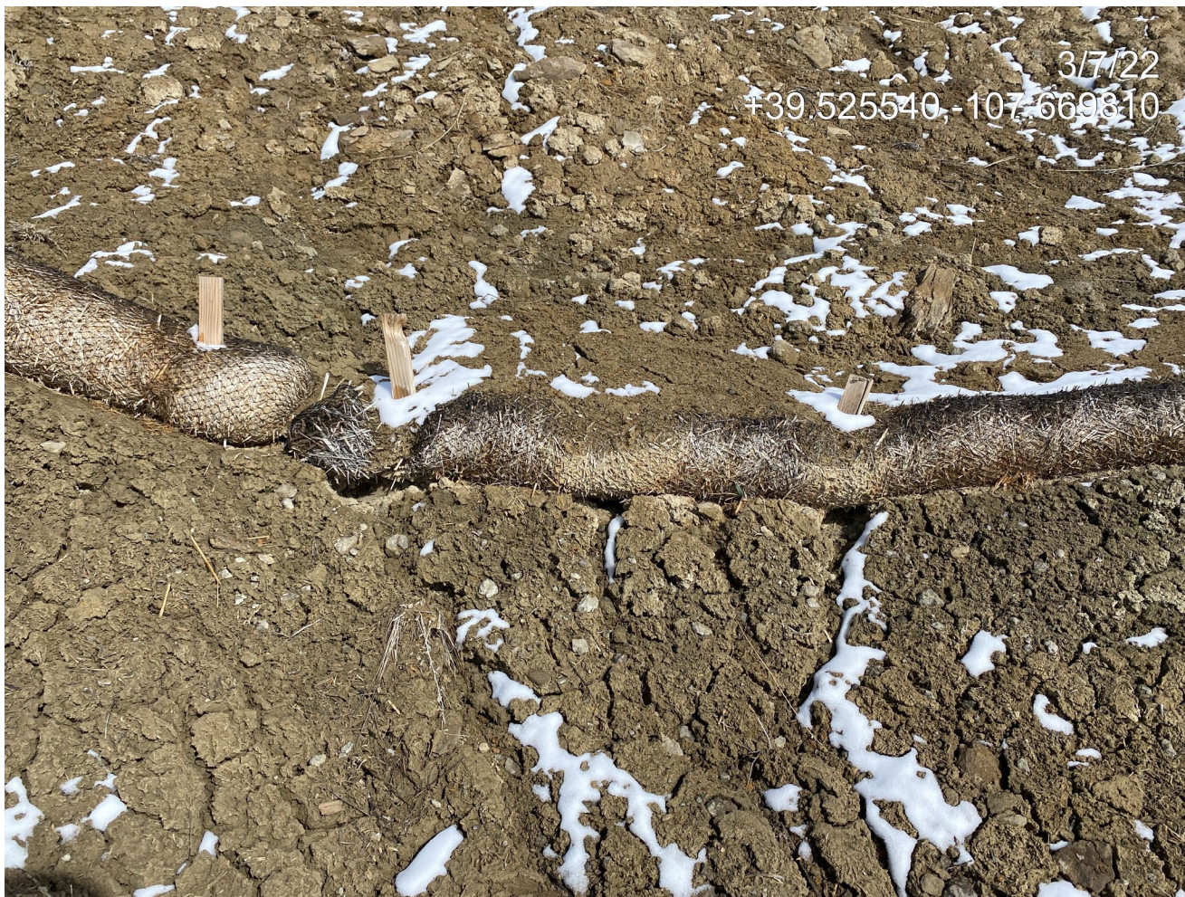
Photo 2. Photo taken from the north of the location shows rill erosion occurring on cut slopes.
