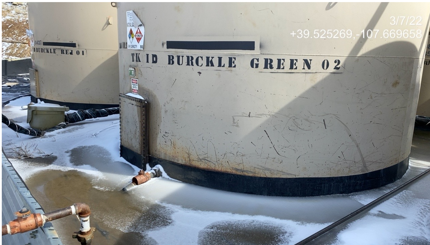
Photo 7. Photo taken from the tank battery shows tank “Burckle Green 02” without a bull plug.
