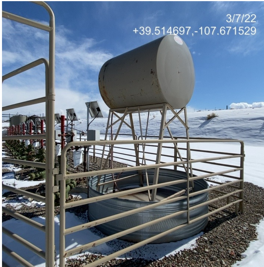
Photo 2. Photo taken from the southwestern production area facing south shows wildlife protection control measures are absent on the stock tank located within the well area.
