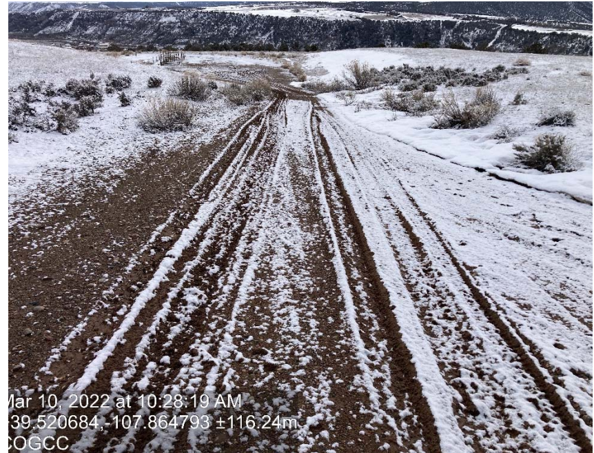
Lack of stabilization/compaction
