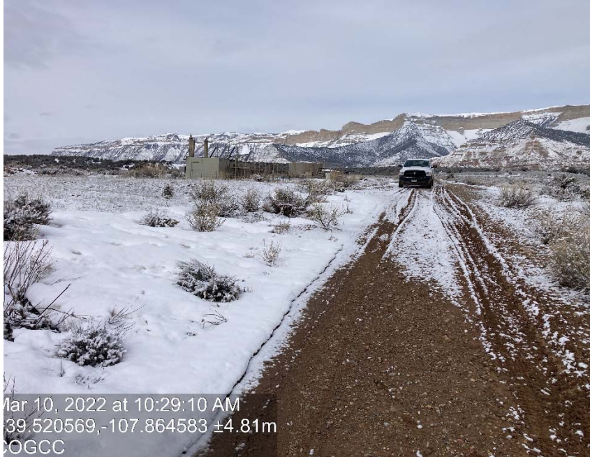
Lack of stabilization/compaction
