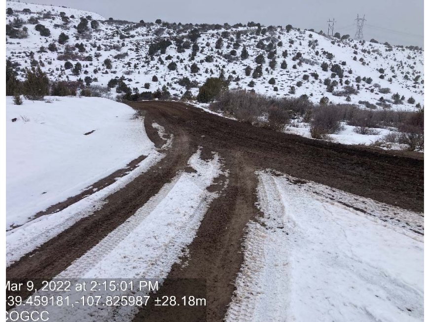
Lack of stabilization/compaction
