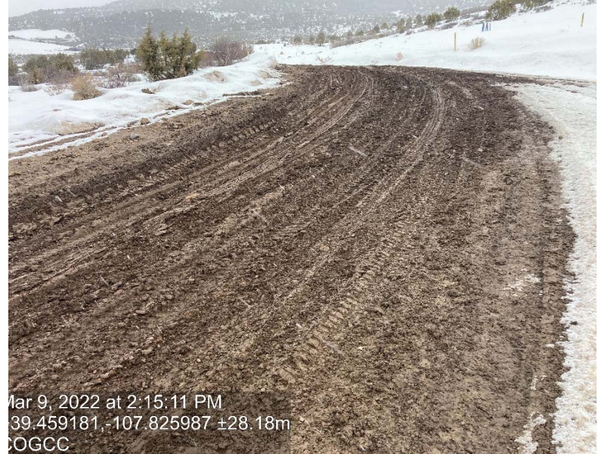
Lack of stabilization/compaction
