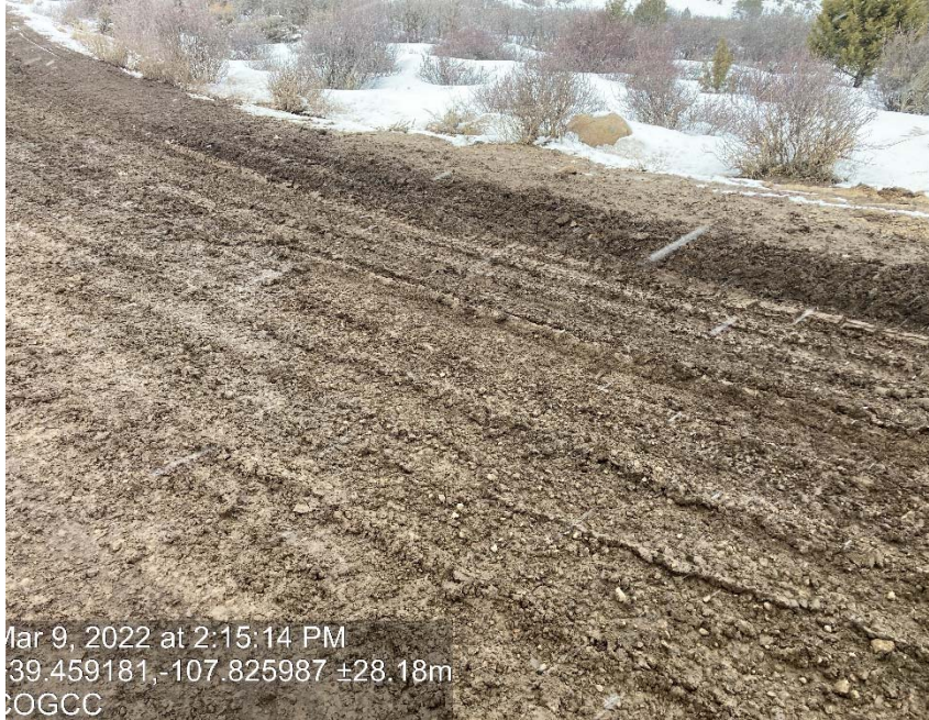
Lack of stabilization/compaction
