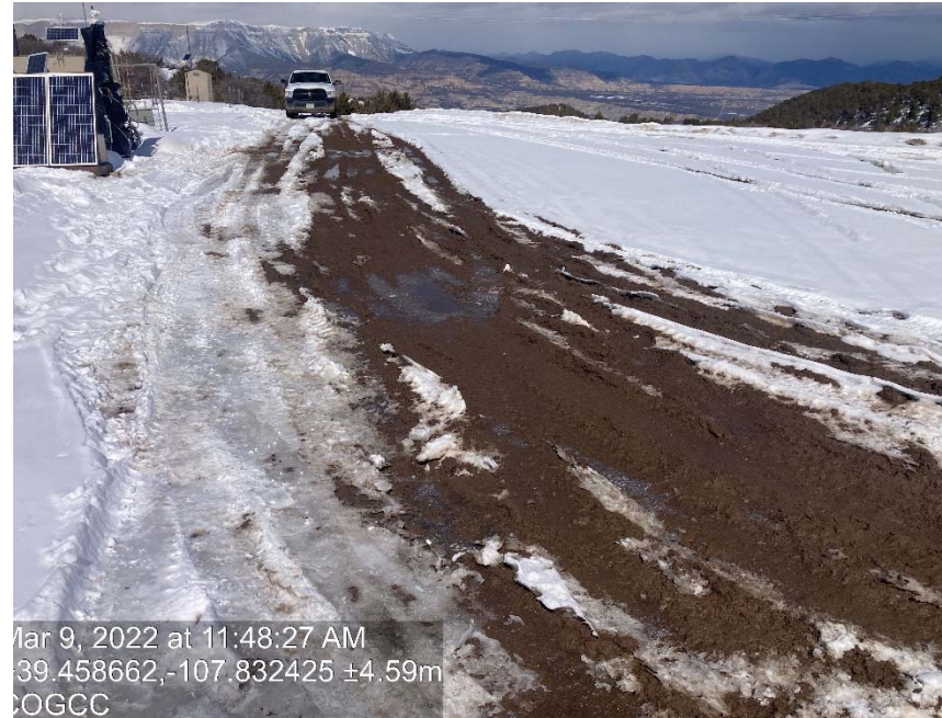
Lack of stabilization/ compaction/ degradation
