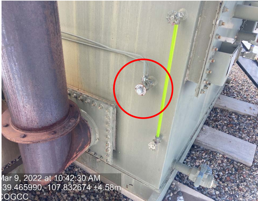
T 12 leaking gas
