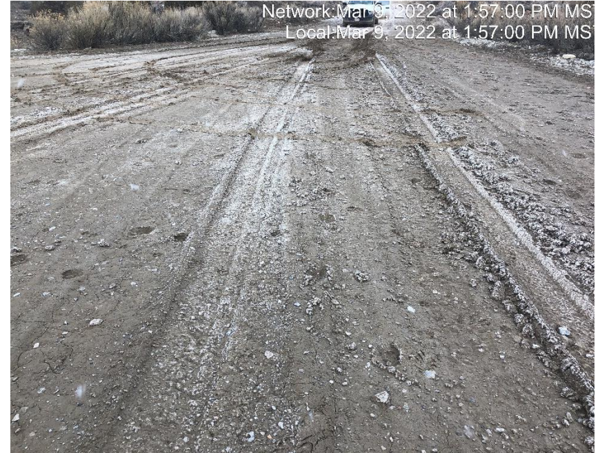
Photo #6125 Insufficient tracking BMP located at entrance to location.
