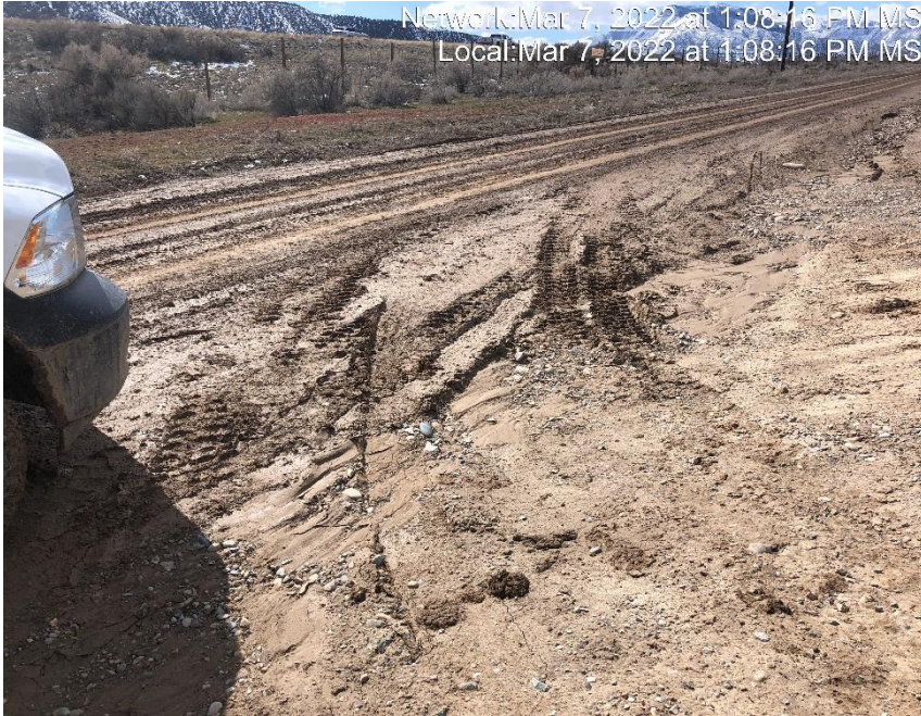
Photo #6115 Insufficient tracking BMP at entrance to location.
