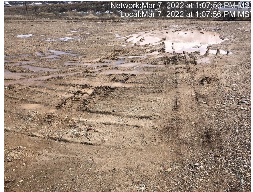
Photo #6114 Location lacks stabilization.
