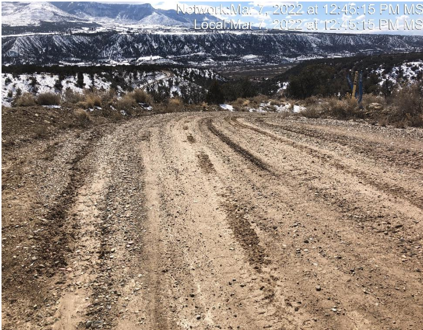
Photo #6110 Insufficient tracking BMP at entrance to location.
