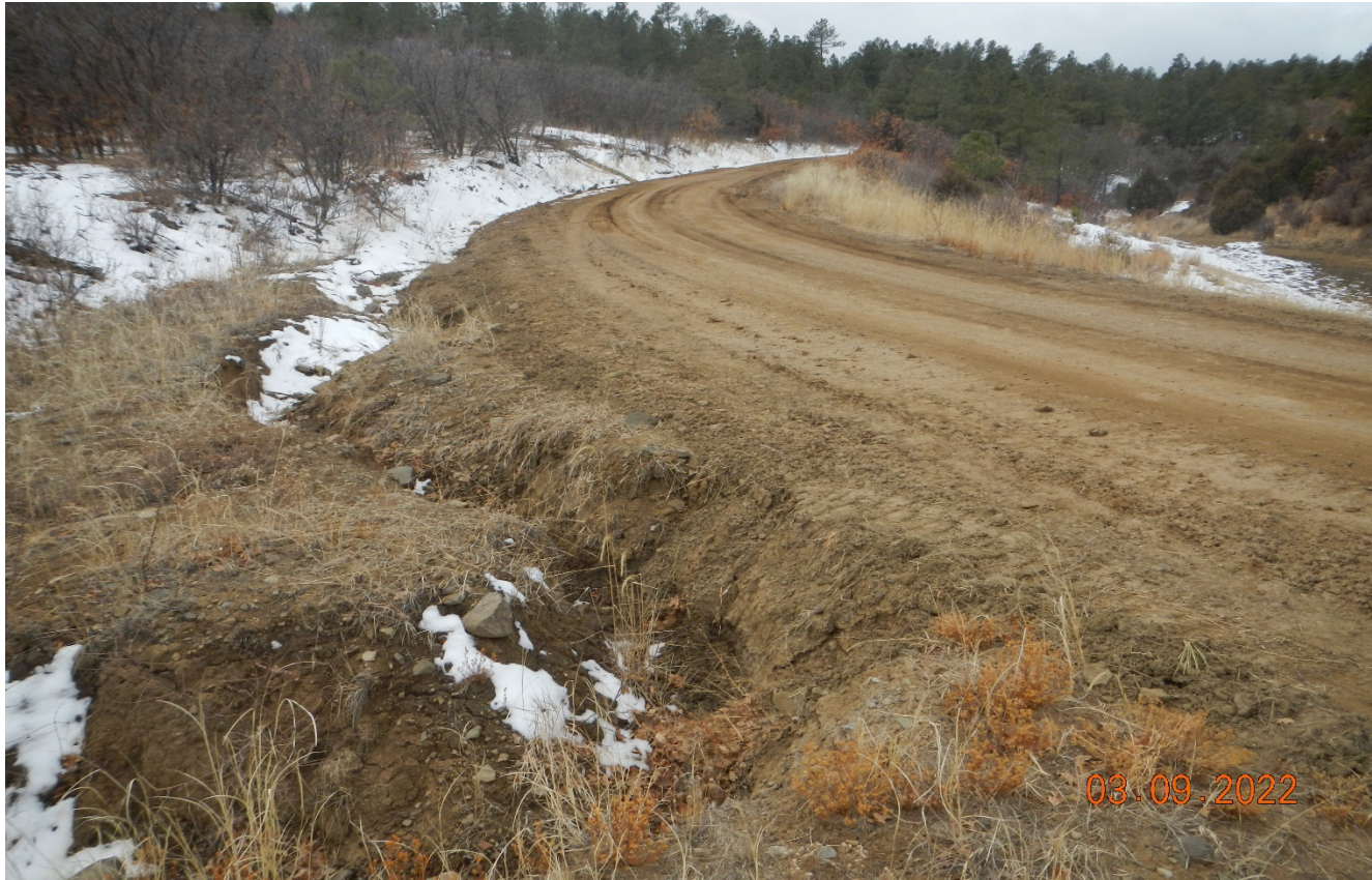
Photo 1. Facing southwest along the main road. Stormwater has caused erosion along the road side. BMP's need to be installed. Lat/Long:37.05530,-104.725025.
