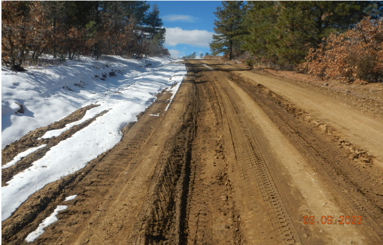
Photo 2. Facing southwest along the main road. There is a lot of vehicle traffic causing rutting of the road. Maintenance and grading of the road will need to be performed.
