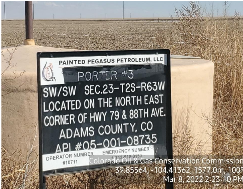
Photo 3: Tank Battery Sign
