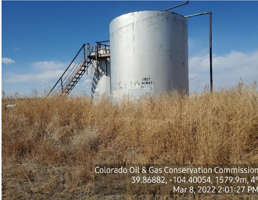
Photo 5: Centralized Tank Battery
