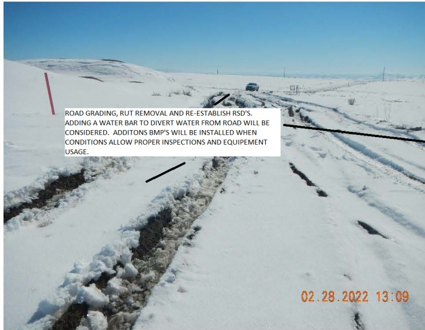
Location lacks compaction/stability
