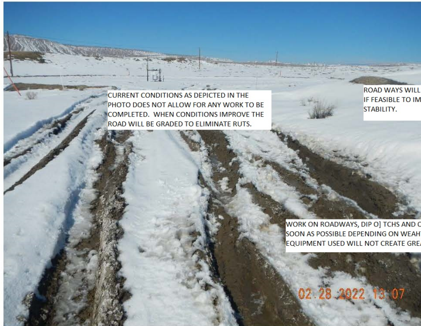
Access road lacks compaction/stability
