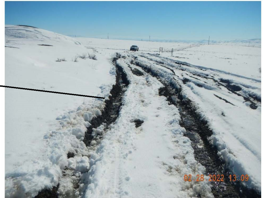
Location lacks compaction/stability
