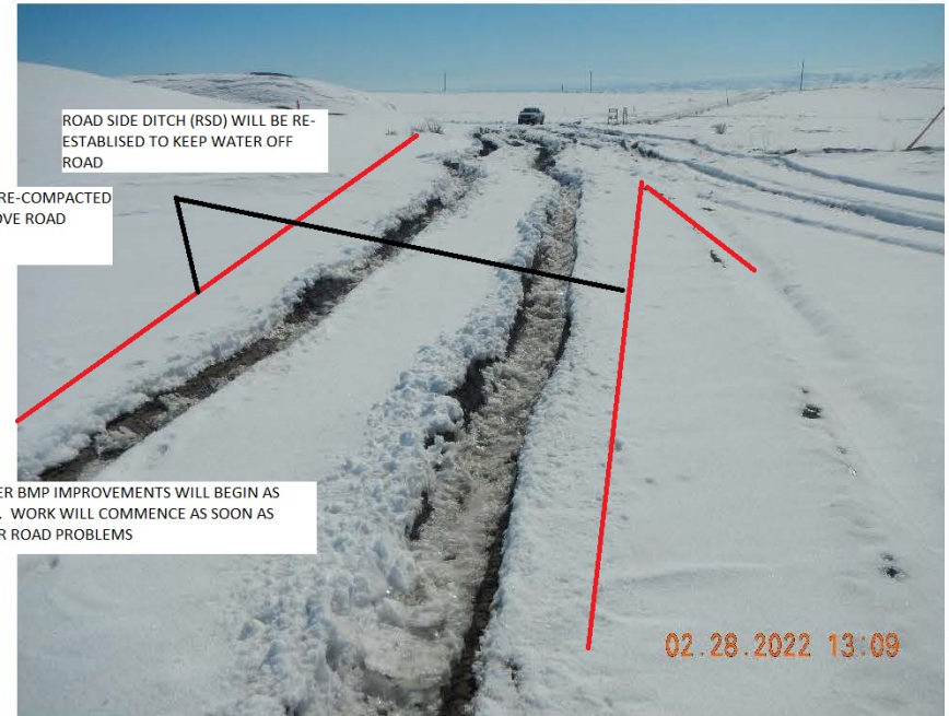
Location lacks compaction/stability
