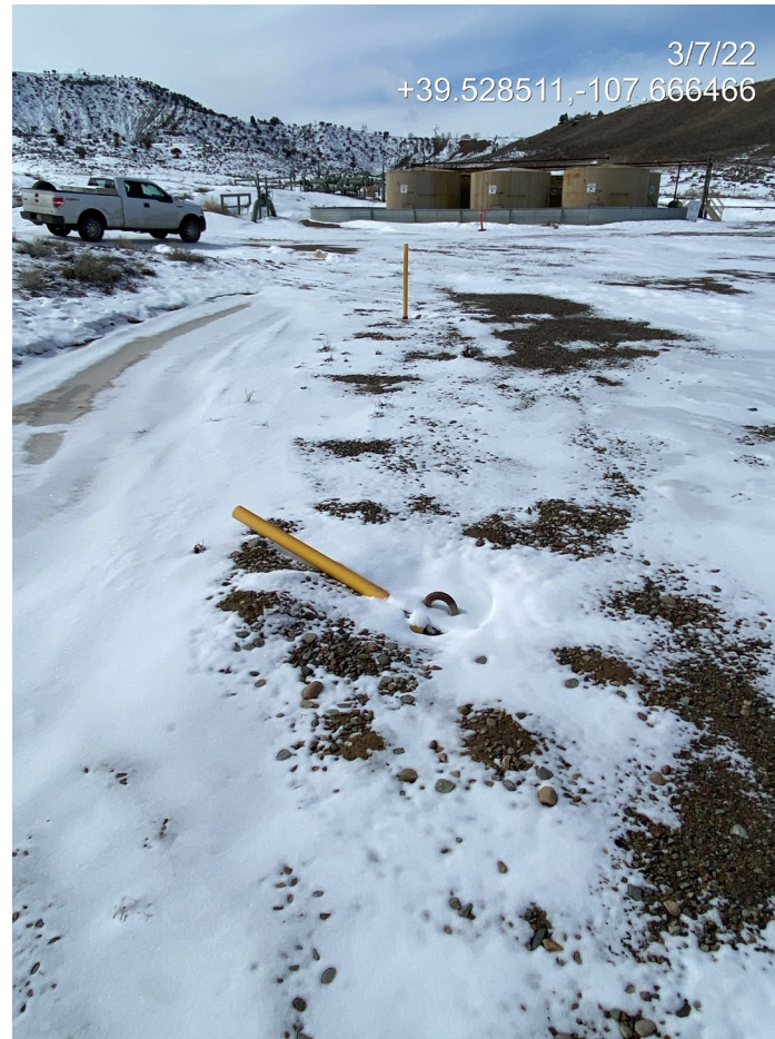
Photo 8. Photo taken at the south of the Location facing southwest shows an anchor marker in disrepair. 3 of 7 counted anchor markers were in disrepair.
