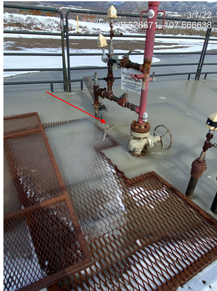
Photo 7. Photo taken at the wells facing north shows well API # 05-045-12060. The arrow points to gas bubbling up in the water indicative of a potential leak.
