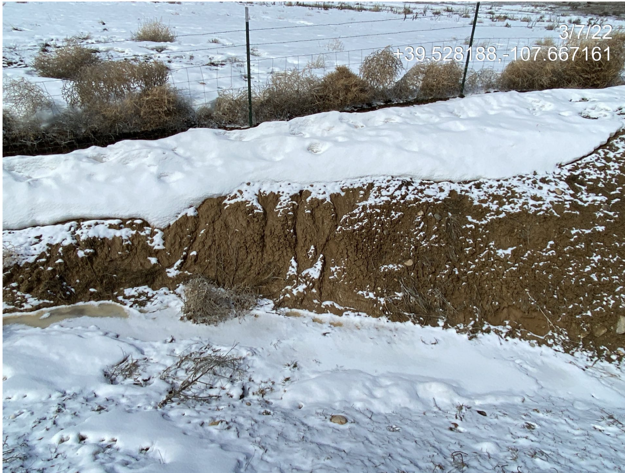
Photo 5. Photo taken at the southwest corner of the pad facing west shows rill erosion occurring on unstabilized slopes of the sediment trap.
