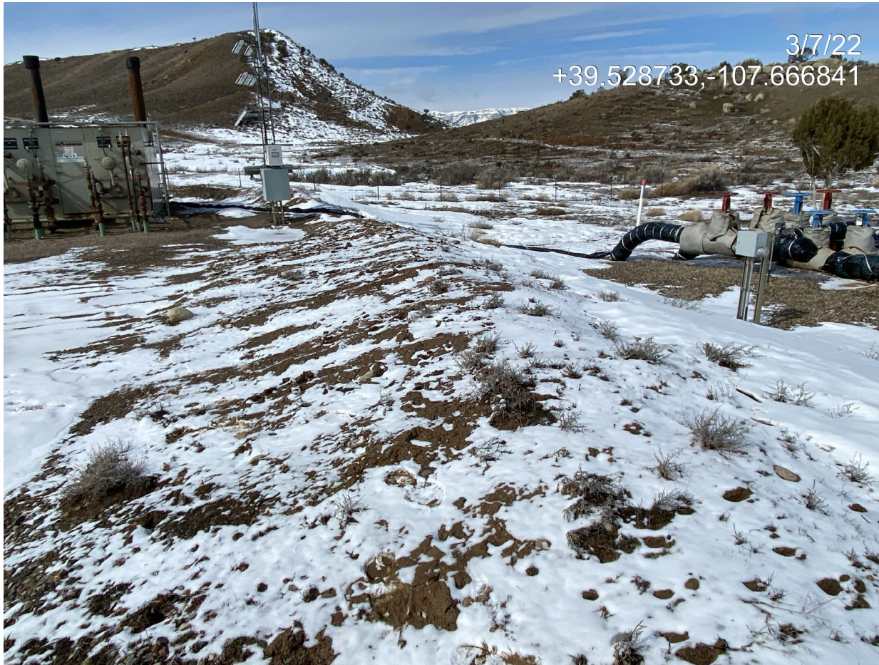
Photo 3. Photo taken at the north of the location facing west shows unstabilized slopes not progressing towards reclamation standards. See additional comments under photo 2.
