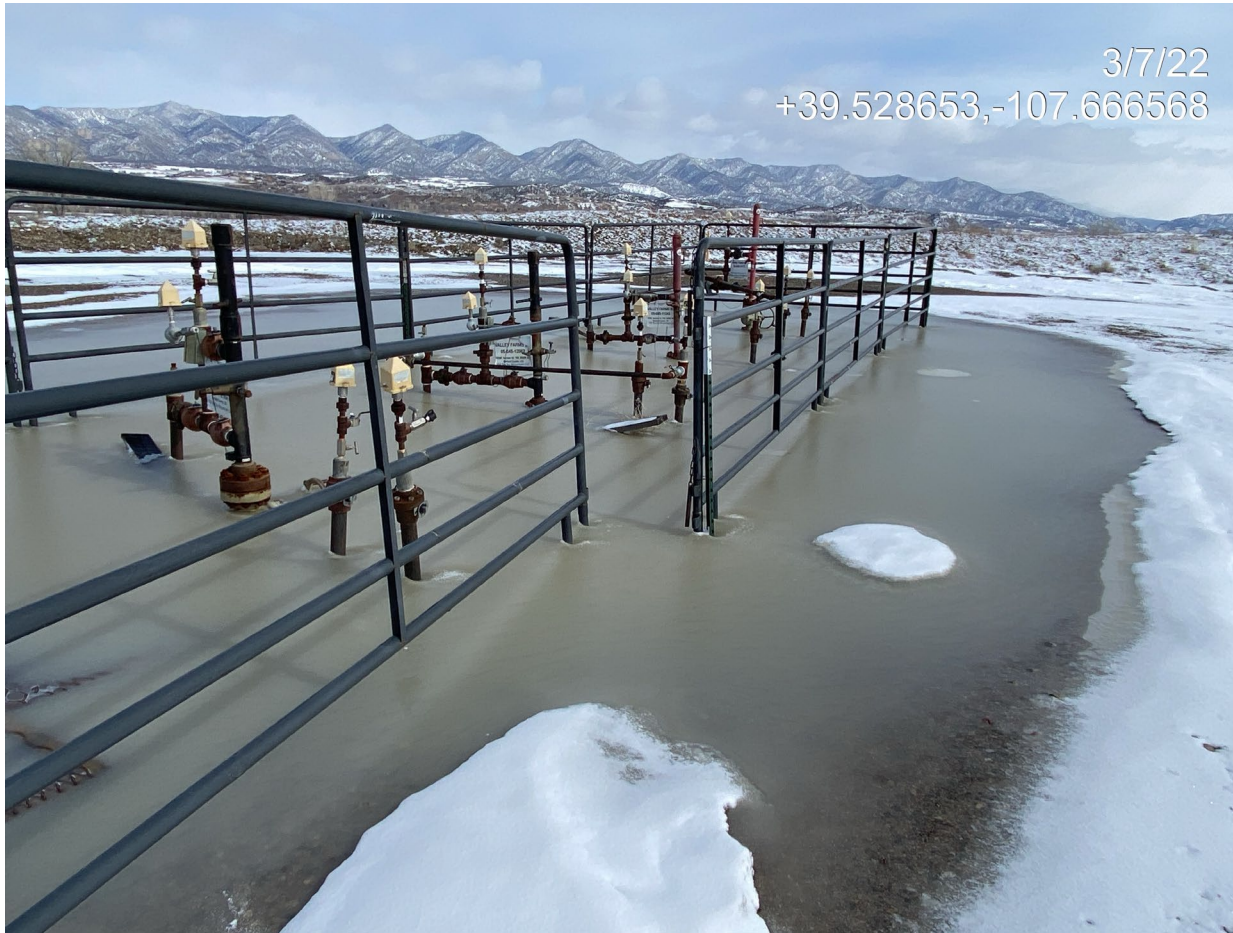
Photo 6. Photo taken at the wells facing northeast shows wells completely inundated with stormwater.
