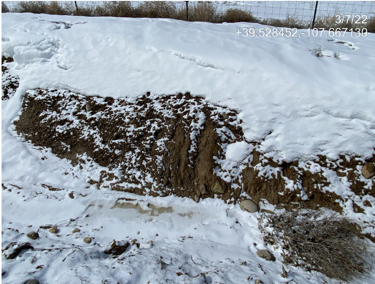
Photo 4. Photo taken at the southwest corner of the pad facing west shows slopes covered in snow. A follow up inspection is necessary to properly asses stormwater management. Exposed slopes show signs of rill erosion.
