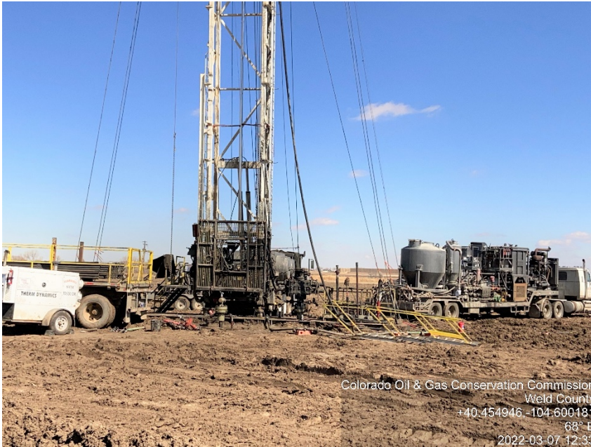
Photo #1 Roth 12-30 (05-123-13046) Wellsite Plugged & Abandoned | PA Plugging Operations: Cementing | WK Final plugs / Cement to surface
