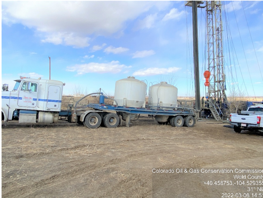
Photo #1 Howard 8-27 (05-123-13326) Wellsite Plugged & Abandoned | PA Plugging Operations Casing stuck
