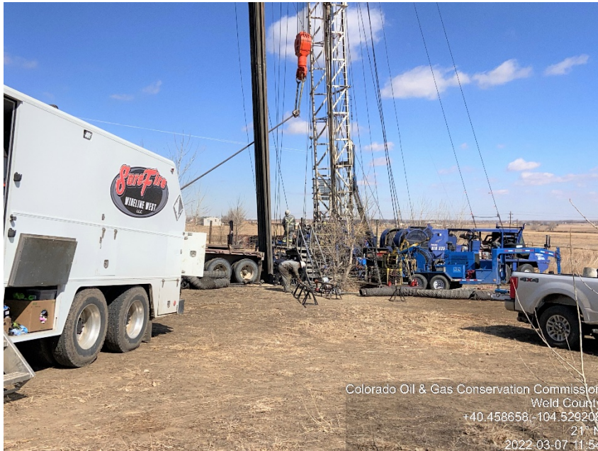
Photo #1 Howard 8-27 (05-123-13326) Wellsite Plugged & Abandoned | PA Plugging Operations Perf for squeeze
