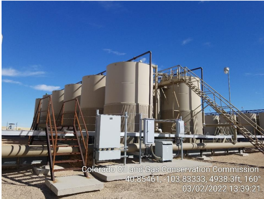
Photo 7 – Produced Water Tanks
