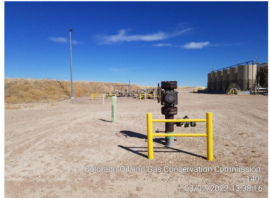
Photo 2 – Unmarked Riser in NW Corner
