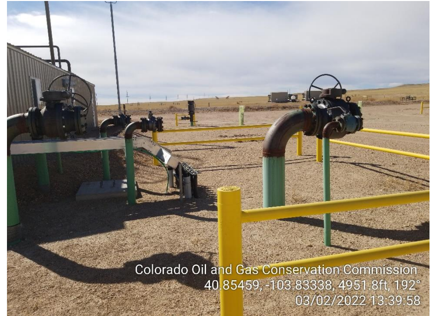
Photo 10 – Unmarked Risers North of Treaters
