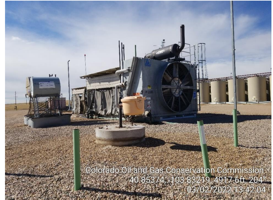
Photo 14 – Compressor – Drain Pit missing Labels
