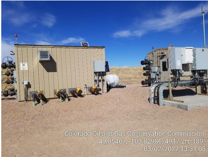
Photo 5 – Gas Lift Injection Meter Sheds
