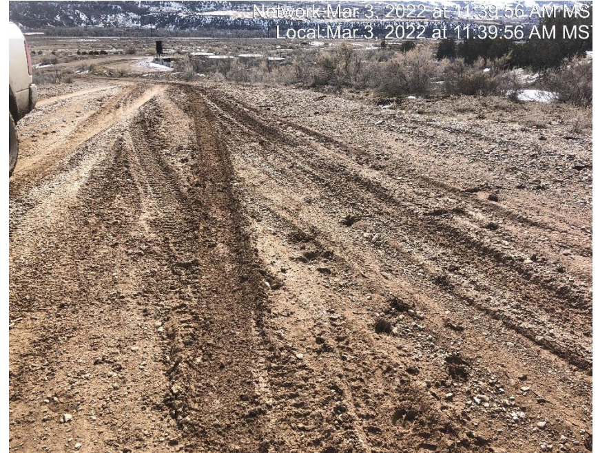
Photo #6079 Insufficient tracking BMP at entrance to location.
