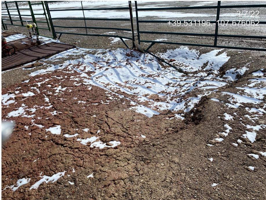
Photo 4. Photo taken of subsidence occurring at dry and abandoned well that has been filled.
