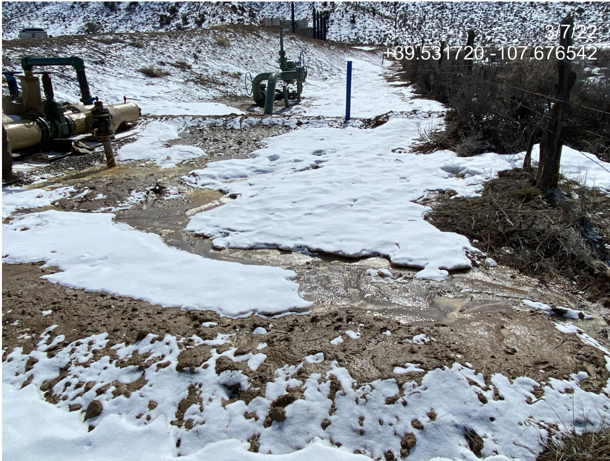
Photo 12. Photo taken from north of the Location facing south. Photo shows the tie in point on a flowline (# 466720) where potentially impacted fluids are flowing around the secondary containment berm and offsite with stormwater runoff.
