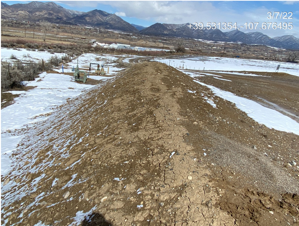
Photo 10. Photo taken from the northeast of the Location facing north showing an unstabilized berm.
