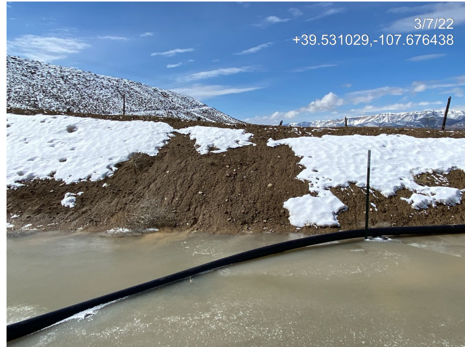
Photo 7. Photo taken from the southwest corner of the Location facing west shows erosion occurring on unprotected slopes.
