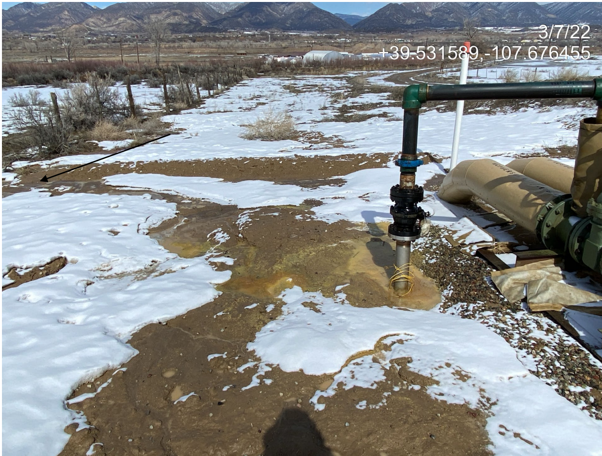
Photo 11. Photo taken from north of the Location facing North. Photo shows an overview of the tie in point on a flowline (# 466720) with potentially impacted fluids accumulating around the tie in point. Note the arrow showing where potentially impacted fluids are flowing around the secondary containment berm and offsite with stormwater runoff.
