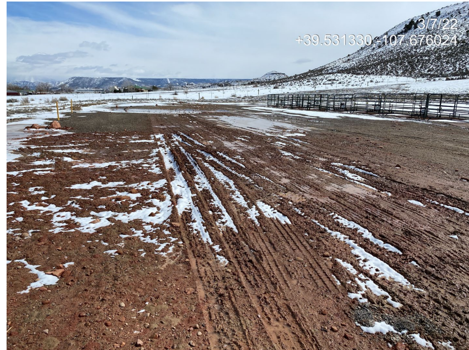
Photo 5. Photo taken at the northwest corner of the Location facing east where sediment from the dry and abandoned well appears to have been dumped on the pad, covering the gravel.
