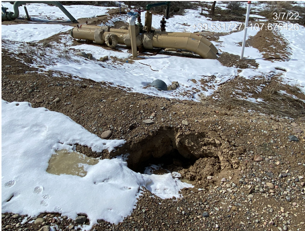
Photo 10. Photo taken from the access road directly north of the Location entrance facing west showing where runoff is cutting into a berm adjacent to a culvert.
