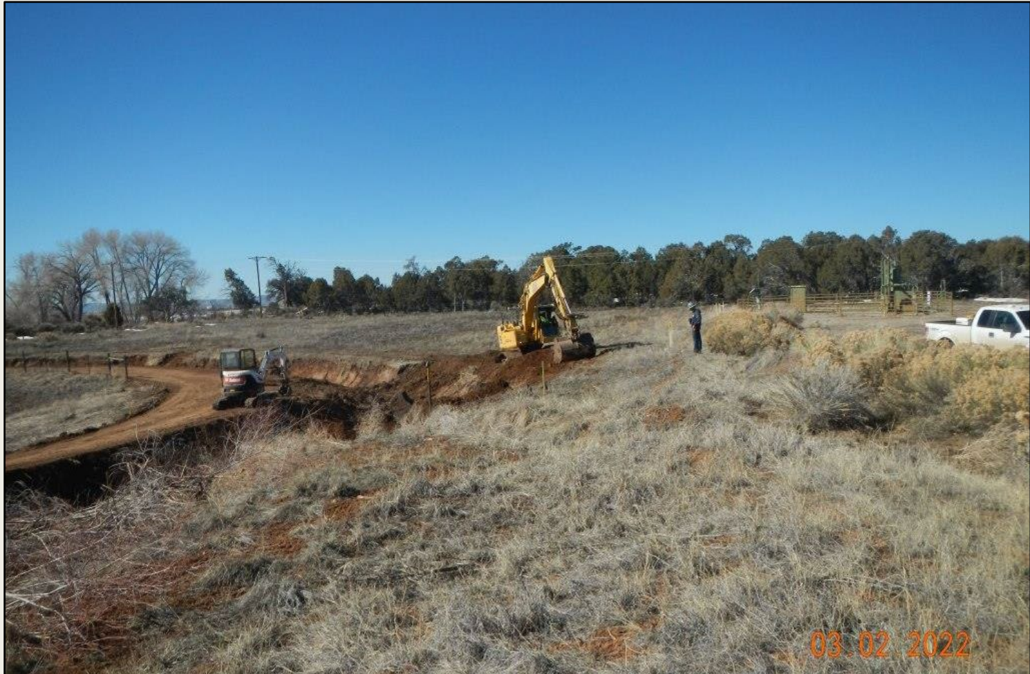
Photo 3. View of the southern project area from the southeastern corner facing westward. Per communication with onsite contractors, excavation work is being conducted by the US Bureau of Reclamation to dredge and maintain irrigation canal that runs adjacent to the southern project area.
