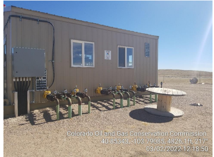
Photo 6 – Gas Lift Injection Meter Shed
