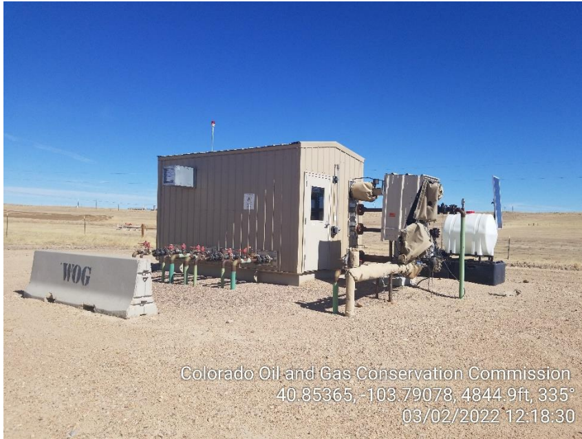
Photo 5 – Gas Lift Injection Meter Shed
