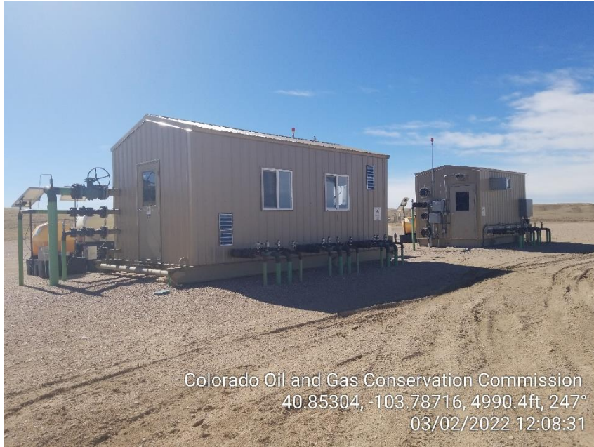
Photo 5 – Gas Lift Injection Meter Sheds
