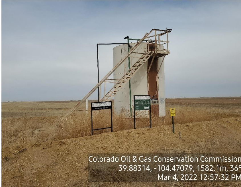
Photo 3: Tank Battery
