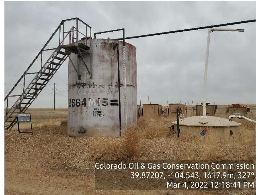
Photo 2: Tank Battery
