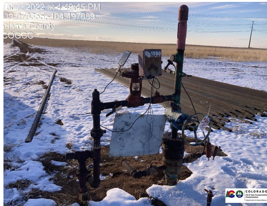
Pic 1 Wellhead. At time of inspection All valves were in close position. LOTO was installed on master valve. Bradenhead is in close position.
