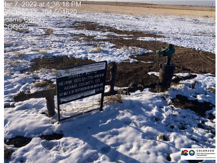
Pic 2 Shively 21-12. At time of inspection all valves were in the close position. During inspection it was observed that gas was leaking out of packing, and Master valve. Valve is in the close position, and will not properly seal. Attempted to tighten hammer union with hammer and would not tighten.
