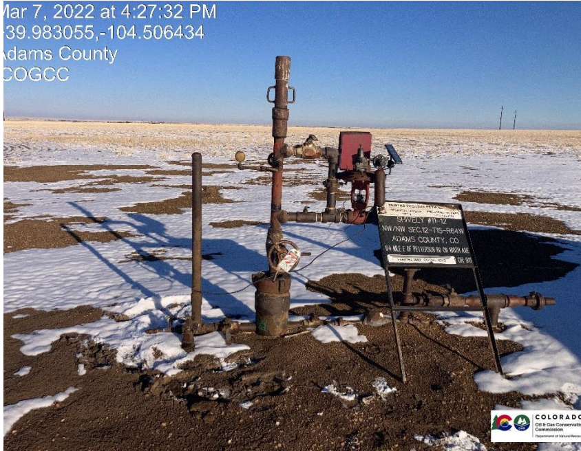
Pic 1 Shively 11-12 wellhead. At time of inspection all valves were in the close position. During inspection well was LOTO.
