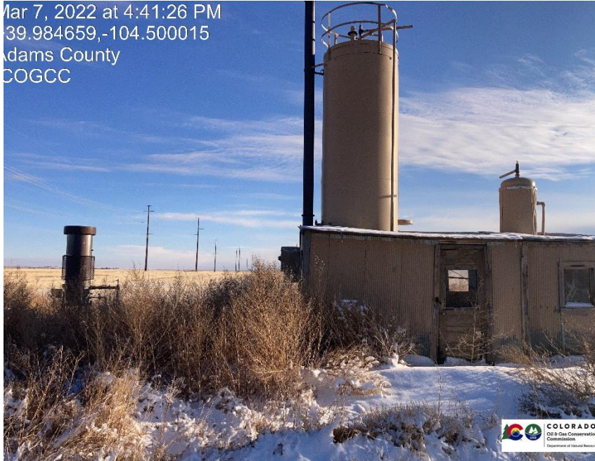
Pic 3 ECD, Separators. Separator house is in disrepair and needs to be removed.
