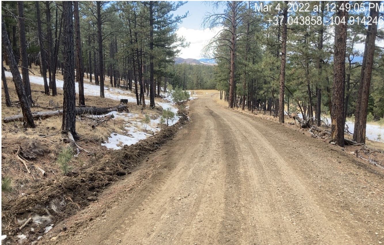
Photo 1. Facing northwest toward the access road.
