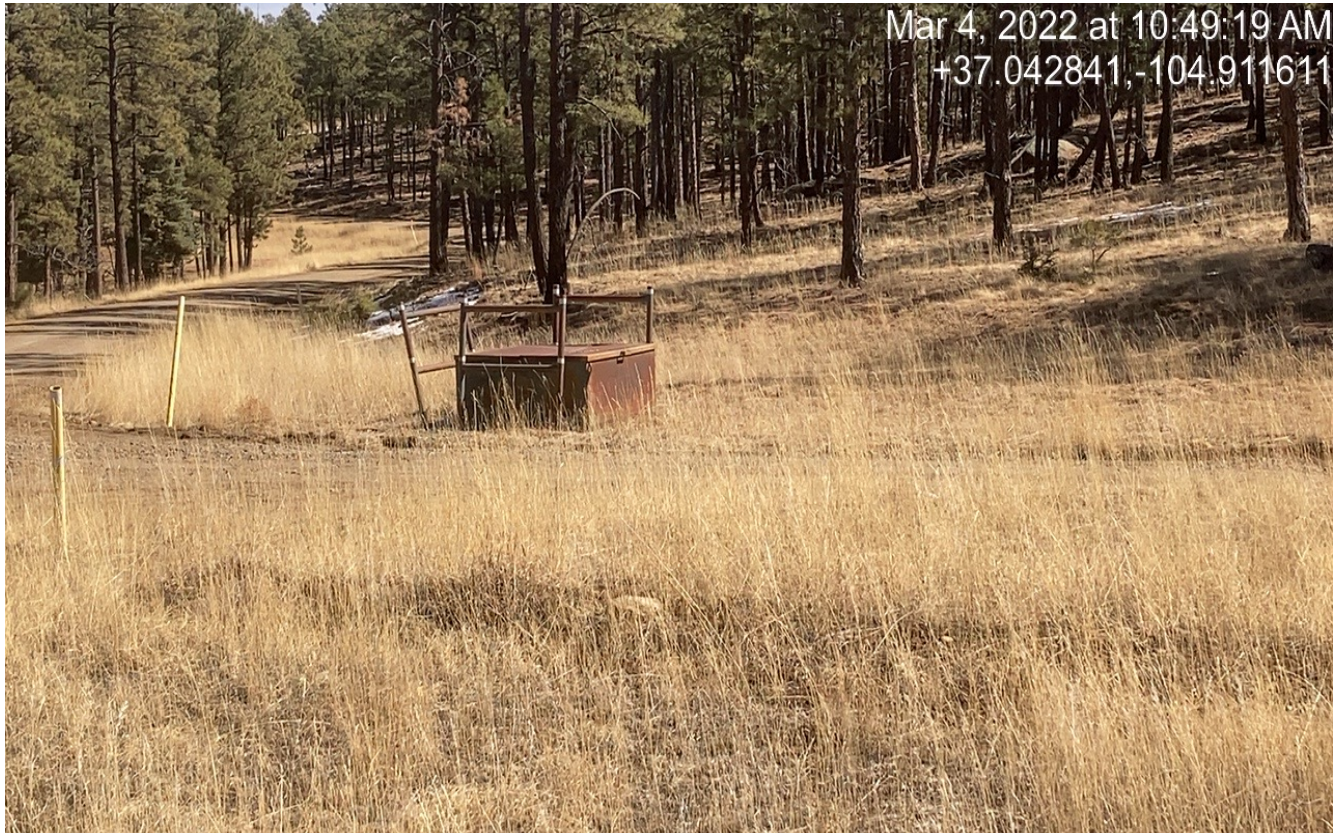
Photo 2. The lid cover is replaced on the valve box.
