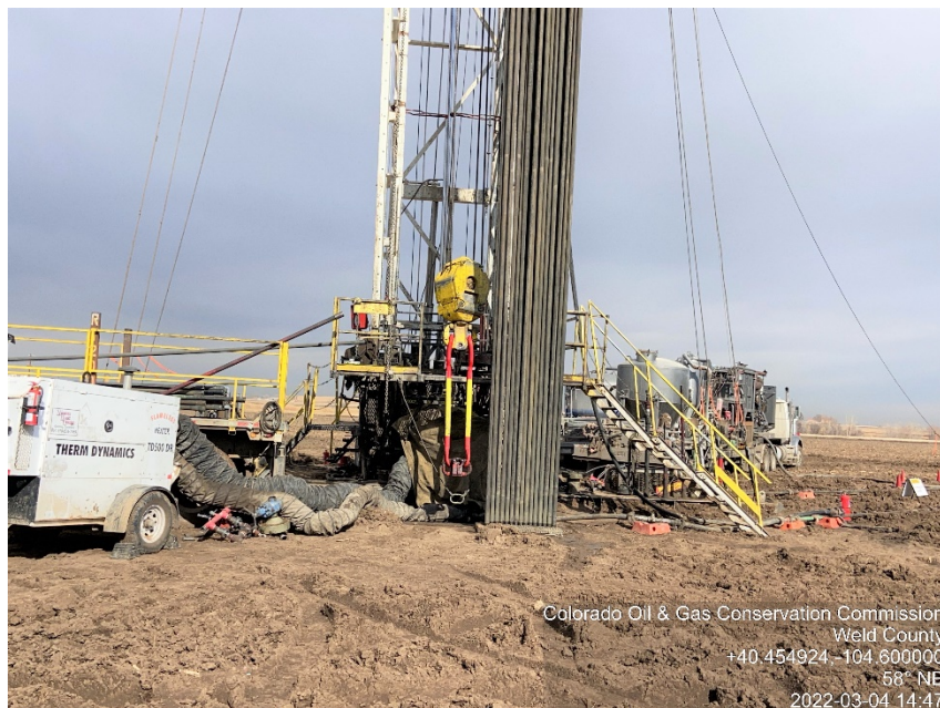
Photo #1 Roth 12-30 (05-123-13046) Wellsite Plugged & Abandoned | PA Plugging Operations: Cementing | WK Intermediate plugs cementing
