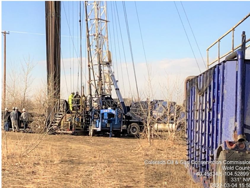
Photo #1 Howard 8-27 (05-123-13326) Wellsite Plugged & Abandoned | PA Plugging Operations Set initial CIBP, prep for squeeze
