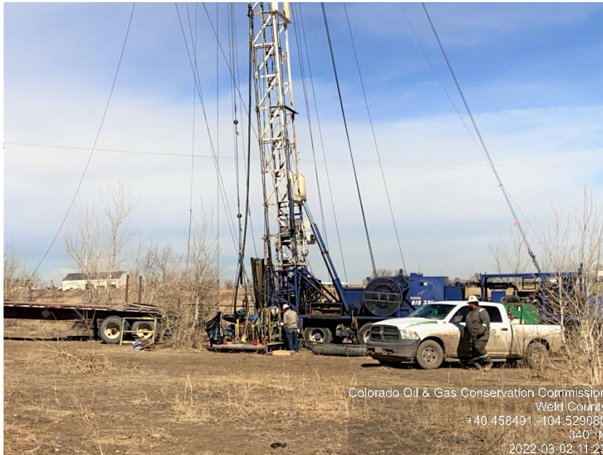
Photo #1 Howard 8-27 (05-123-13326) Wellsite Shut-In | SI Plugging Operations: Bleed down | WK Pump mud to kill well, prep for plugging.
