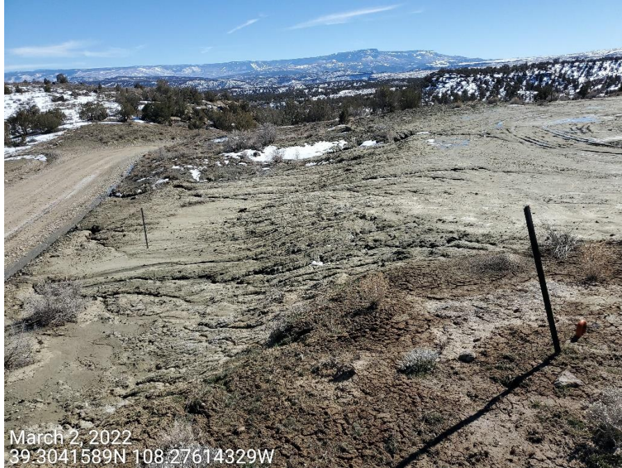
Photo 6: Photos taken from the east end of the Location, facing south. Photo left dated 3/2/2022; photo right dated 7/26/2021. Photos show erosion degradation due to runoff from the location has continued since the previous inspection; control measures to manage runoff and minimize erosion degradation remain missing or insufficient on the Location.
