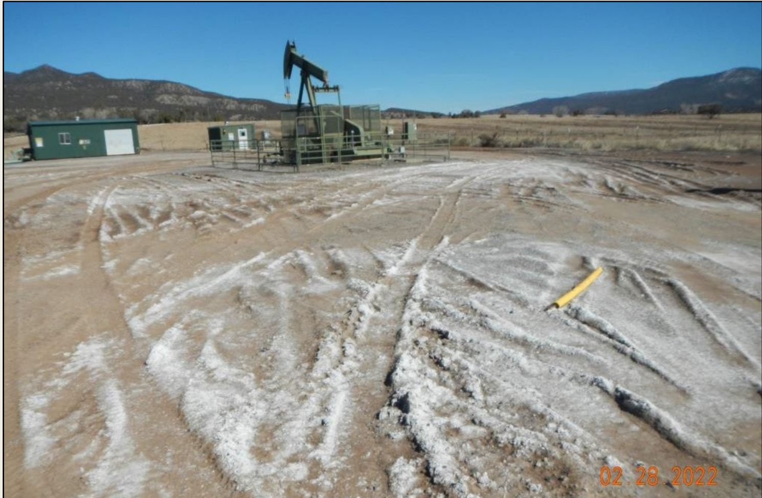
Photo 1. View of project area from the well pad entrance facing center. Significant salt crust observed on the well pad surface.
