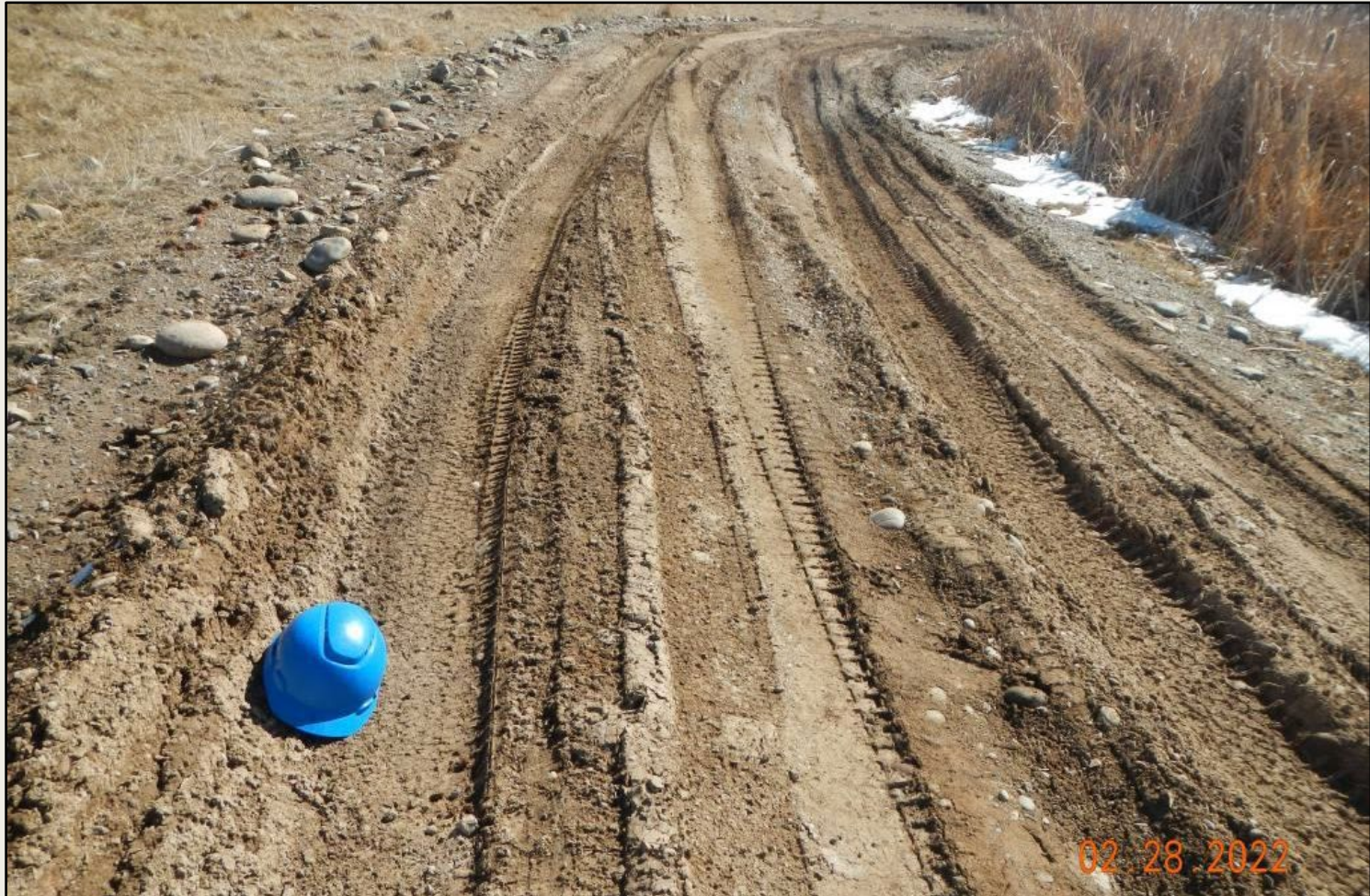
Photo 5. View of deep rutting up to 18 inches deep, observed on the access road, needing stabilization. Hard hat in place for scale.
