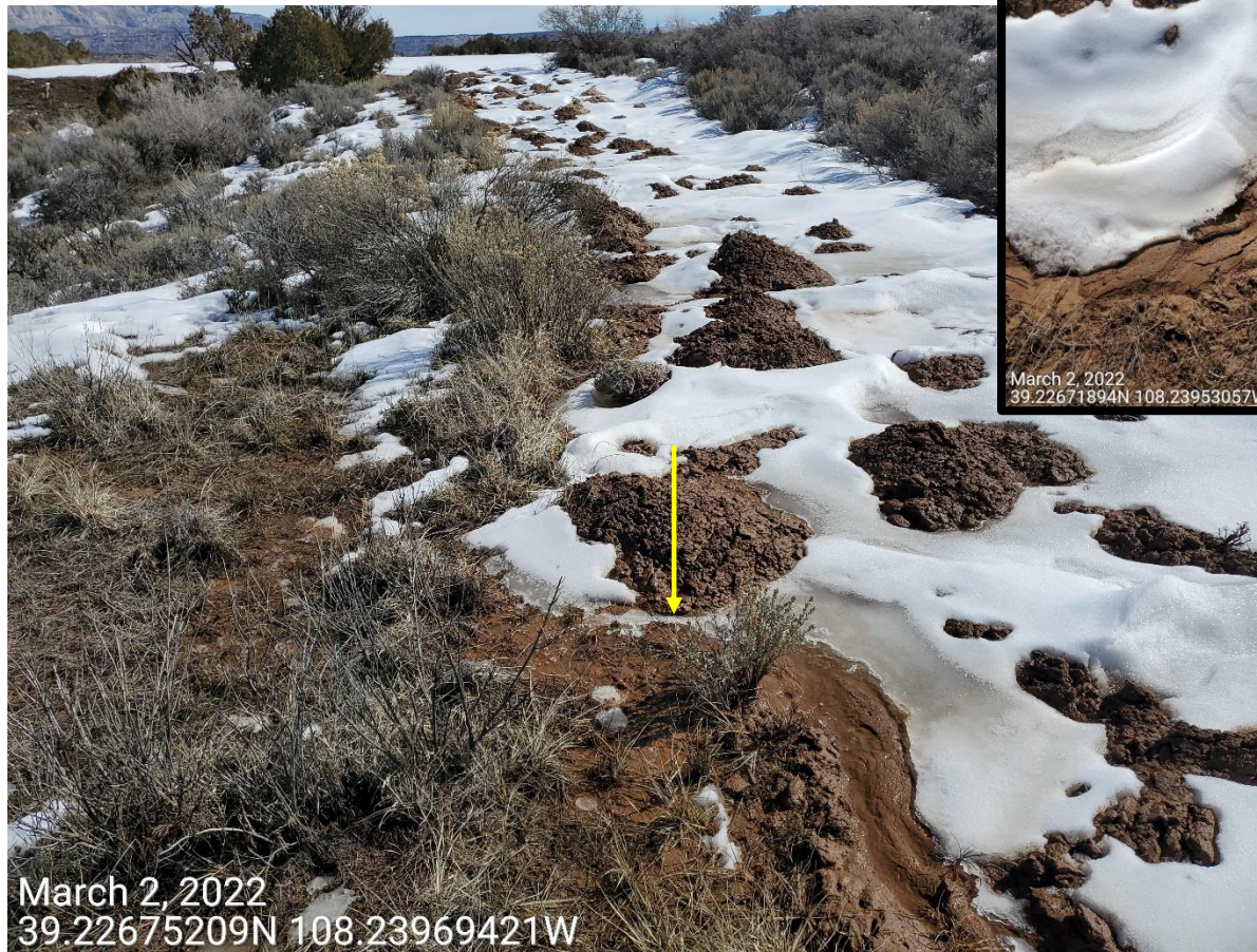
Photo 3: Continued from photo 2. Photo shows Operator has “pot-holed” the access road. Photos show sediment transport and deposition observed to do unstabilized soils at access road.
