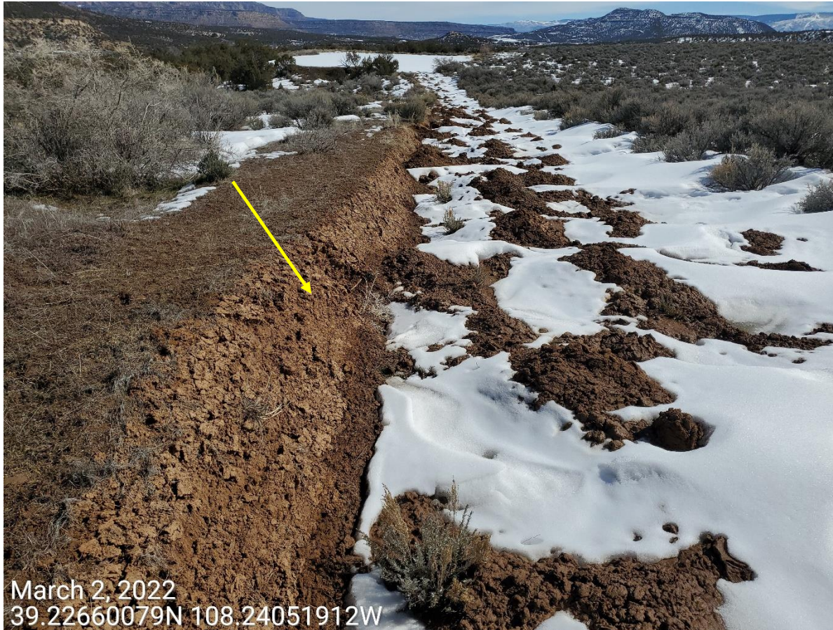
Photo 1: Photo taken from the access road, facing east. Photo taken from the access road. Photo example showing access road has not been recontoured/regraded/reclaimed in accordance with 1004 rules.
