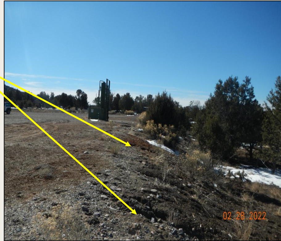
Photos 4/5. View of erosional rilling observed within the western fill slope (multiple areas). Stabilization is needed here.
