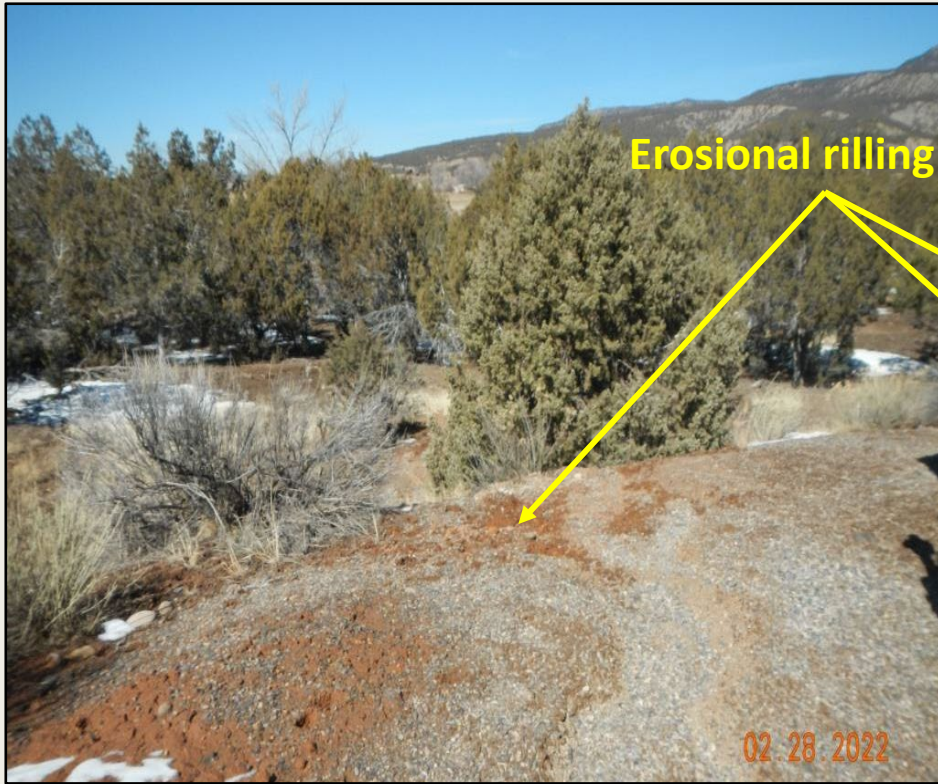
Photos 4/5. View of erosional rilling observed within the western fill slope (multiple areas). Stabilization is needed here.
