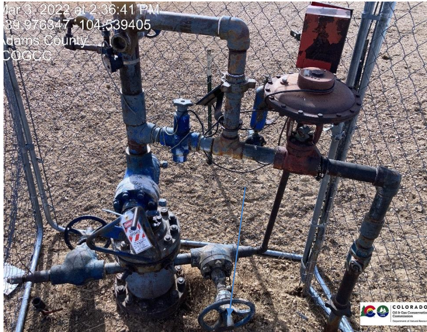
Pic 1 wellhead, At time of inspection master valve, flowline valves, and casing valves were in close position. 1 casing valve appears to be seized in the open position. Bradenhead valve is closed.
