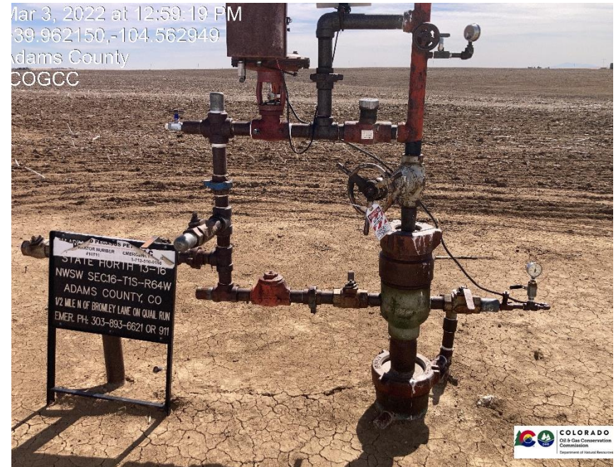
State Horth 13-16. At time of inspection casing valves and master valve were in the open position. During inspection master valve, and
